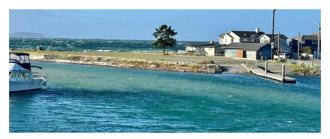
The picture above was taken on November 2<sup>nd</sup>, during our first big wind event from the west. You can see the plume of sand entering the siltation basin as the waves pounded the beachfront to the north of the jetty canal. These events are the cause for us to require maintenance dredging of the basin. On a normal day the water could be crystal clear coming into the canal. But these big storms have the energy to move a lot of material and the incoming tides bring it all right in.
