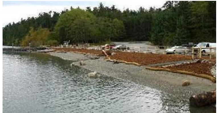
Cornet Bay soft bulkhead project
